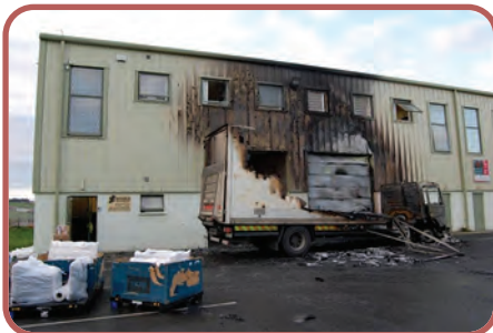
'Explosion' of debris from both sides and top of vehicle – fireball projected onto building cladding.
