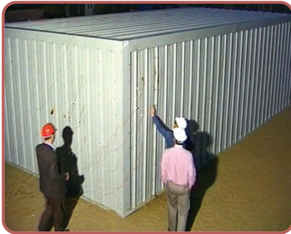
Figure 16. Fully instrumented test building
