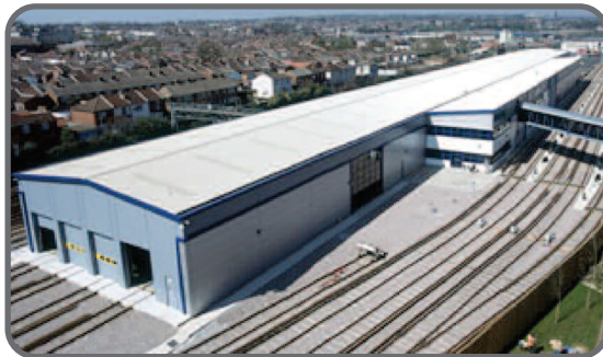
External roof panel application
