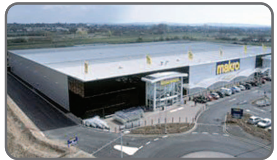
External: roof and walls
