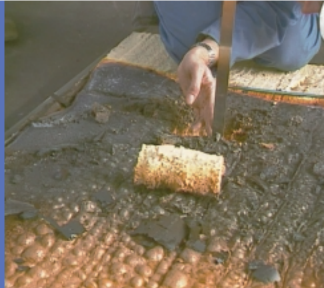
Site assembled built-up systems
