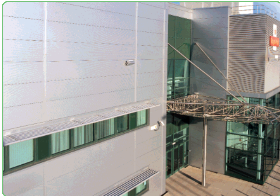
Figure 10. Built in compliance using insulated panels. Insulated panels have the benefit of a guaranteed U-value and computer 'ψ' and 'f' values to confirm compliance. Factory engineered joint details restrict air leakage to a minimum.
