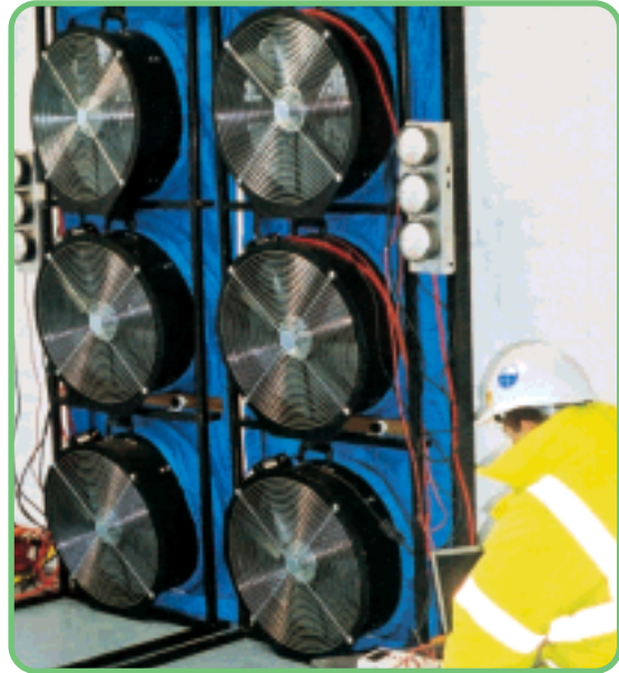
Figure 3. Air pressurisation testing equipment
