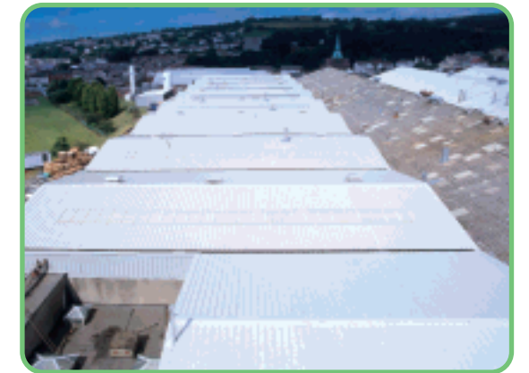
The pictures illustrate before and after refurbishment with insulated panels
